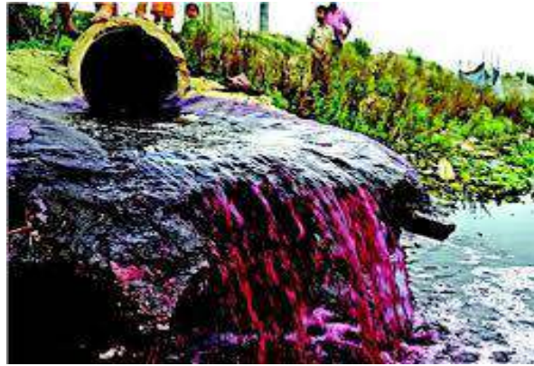
Fig 7: Chemical colour in drainage
